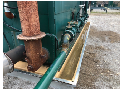
EQUIPMENTGUARD pads elevate equipment so flame arrester piping can pass safely over the low-profile containment wall and prevent exposure to standing rainwater
